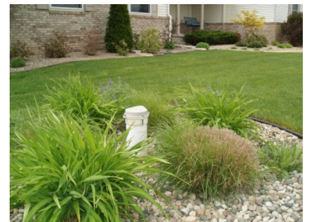
Attractive landscaping protects a 12-inch high wellhead.
